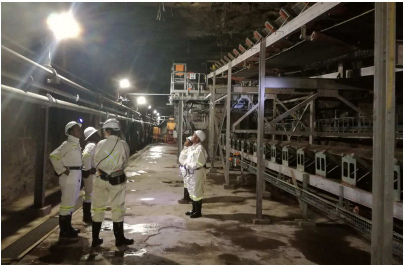
South Africa. 2011. Kalagadi Manganese Mine © 2017. African Development Bank Group
