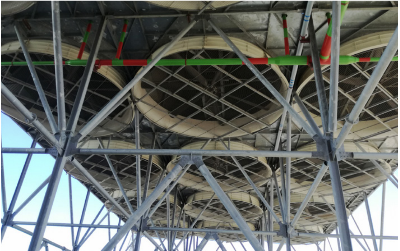
South Africa. 2015. Xina Solar Plant © 2017. African Development Bank Group
