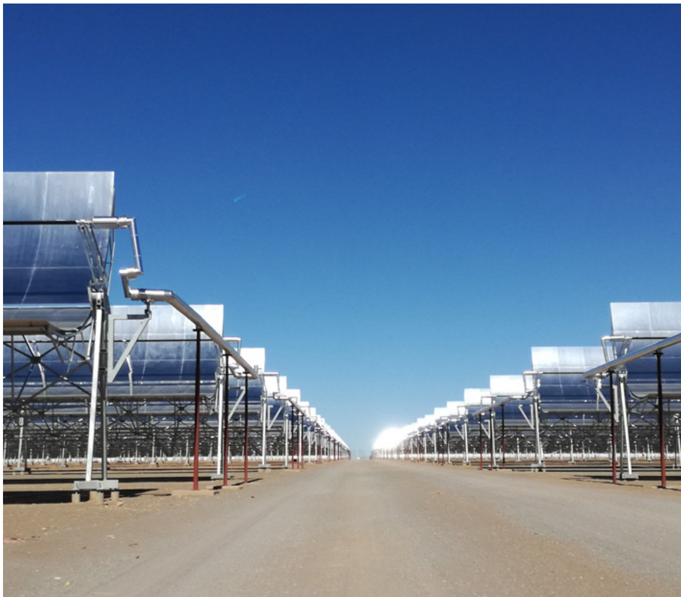
South Africa. 2015. Xina Solar Plant © 2017. African Development Bank Group
