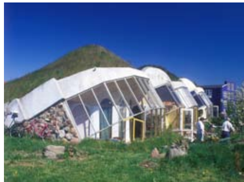
© Martin Bond / Still Pictures Ecological houses at eco-village with earth sheltering (at rear), turf roofs and various active & passive solar features. Dyssekilde, near Hundestad. Denmark.
