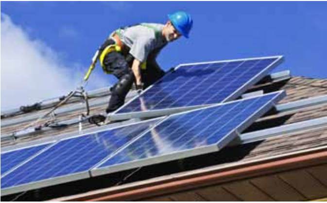
Illustration 10. Solar Photovoltaic installer with safety gear
