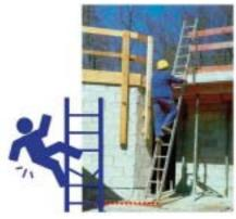
The use of fixed ladders, mobile ladders, suspended ladders, extension ladders and access ladders is subject to certain regulations. All must provide firm grip and secure footing. Carrying even light and manageable loads up or down ladders should be avoided wherever possible.
