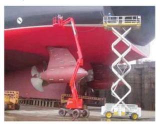
Elevating platforms should be chosen according to the type of work to be carried out and after a detailed analysis of surrounding environment.
